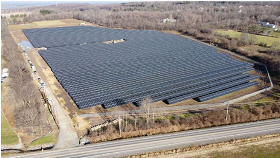
Novis Renewables' North Eagle Village Solar Farm in Manlius (NY, USA)
