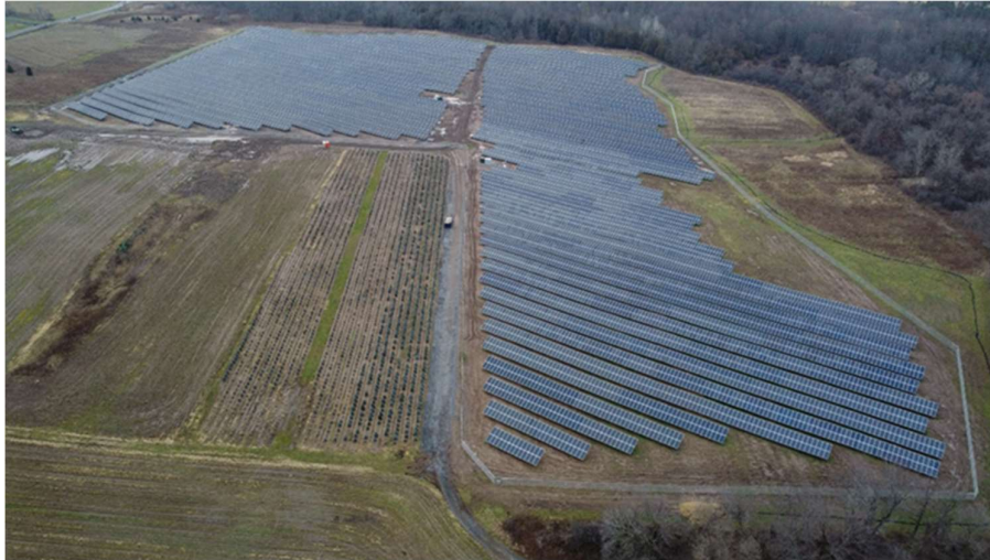
Novis Renewables' Green Lakes Solar Farm in Manlius (NY, USA)
