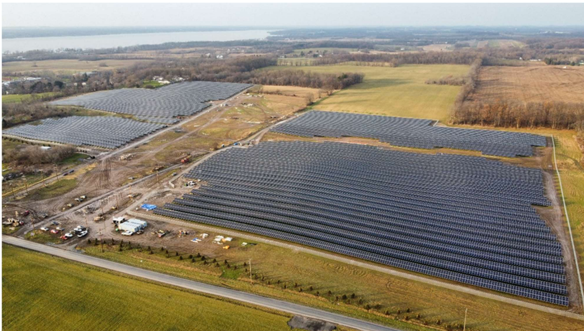
Novis Renewables' USA 963 and USA 40 Solar Plant (NY, USA)
