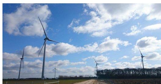
The plant consists of five Enercon E92 wind turbines and has an installed capacity of 11.75MW, generating approximately 27,000 MWh annually. The renewable energy produced is the equivalent to the energy consumed by 7,000 homes and will save almost 12,000 tonnes of CO2 per year.
